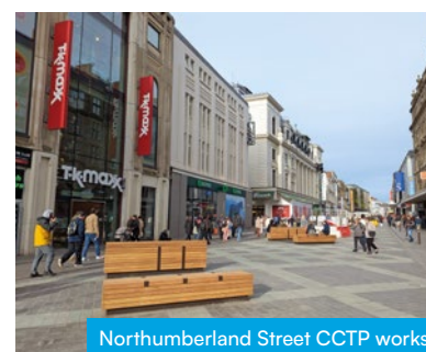
Northumberland Street CCTP works
