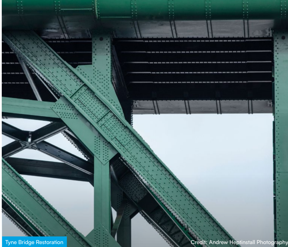
Tyne Bridge Restoration
